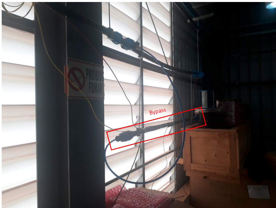
Figure 5.3 – Bypassing the pipe to take measurements directly in a hole in the pipe.
