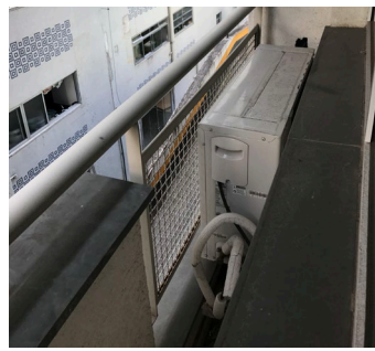
b) Balcony used as service area to house the condenser unit
