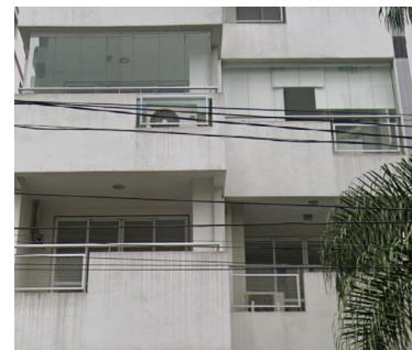
c) Office building façade with condenser unit in the balcony
