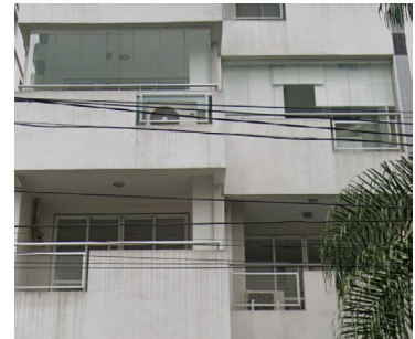
f) Office building façade with condenser unit in the balcony
