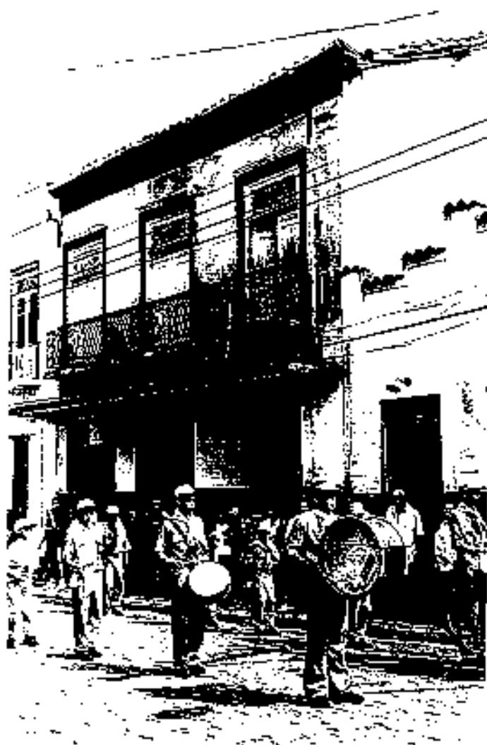
II. 742. Rua Manoel de Aguiar, s/n
