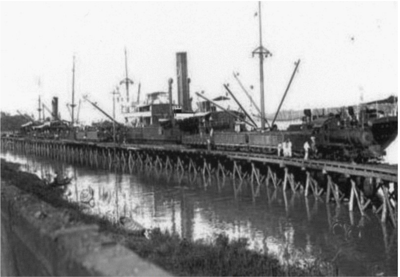
The ss Holland on the jetty in Porto Velho.
