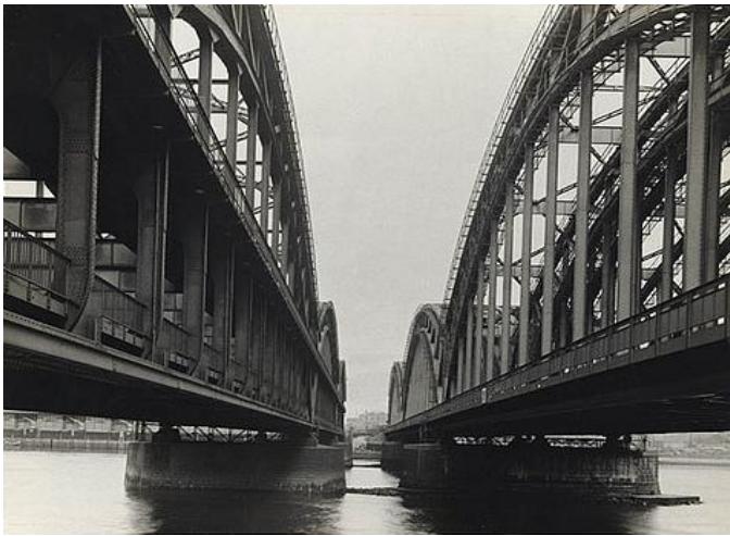
Figura 12: Albert Renger-Patzsch, Railroad bridge , 1927.
