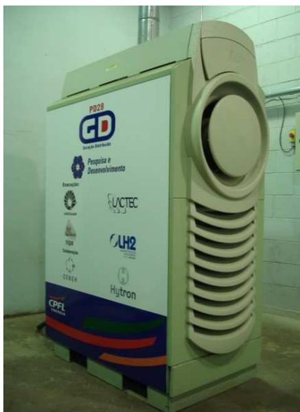
Figura 4.2 - Microturbina Capstone 30 kW
