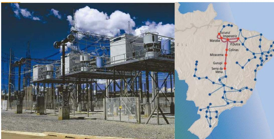
Figura 3.15: TCSC – Serra da Mesa, 550 kV, 107.46 MVar– Figura Manual SIEMENS PTD
