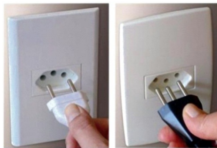
Figure 4 – Brazilian plugs and outlets as required by the standard NBR 14136
