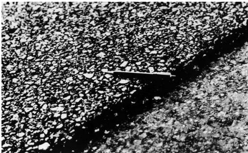
Figura 3.11 - Camada de Porous Friction Course – PFC (FAA, 1997)
