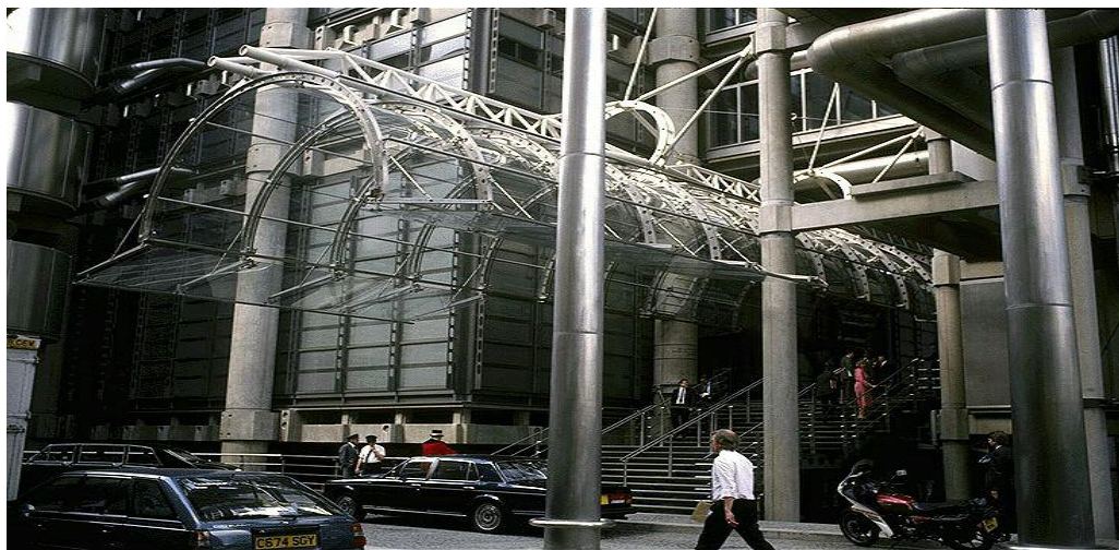
Figura - 4.1.1- Lloyds Building
