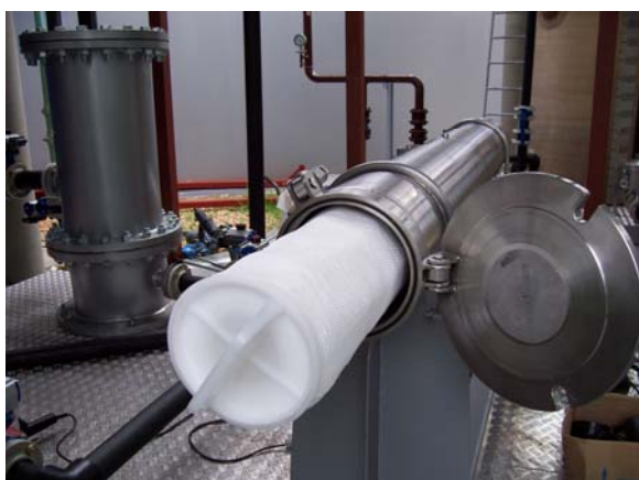
Fig 5.13 – Filtro Cuno high flow filter
