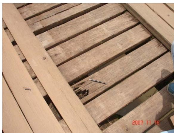
**Figura 6.53 – Tábua deteriorada**
